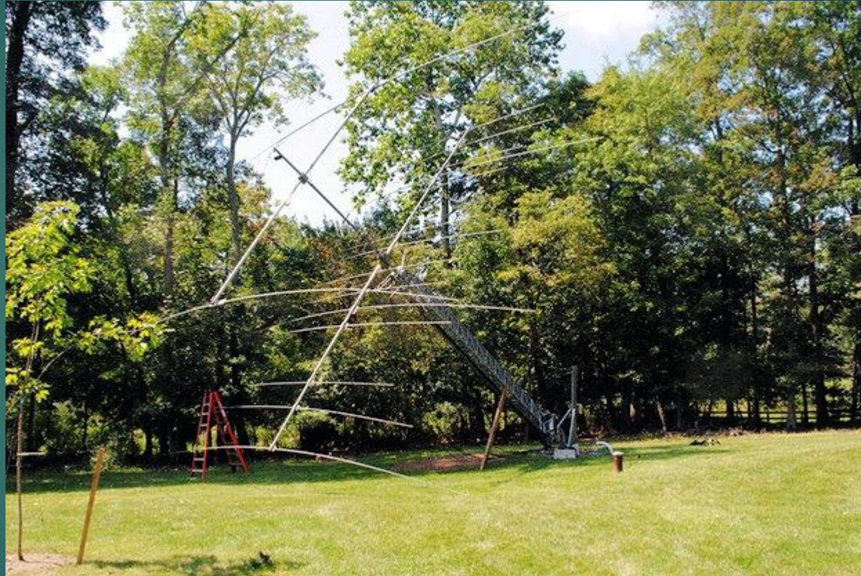
Tower Partially Tipped to Adjust Elements for SO2R in 2015
