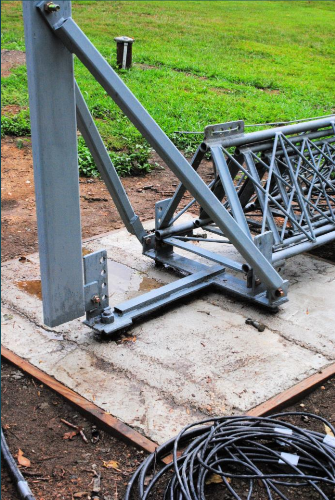
Tower Partially Tipped to Adjust Elements for SO2R in 2015
