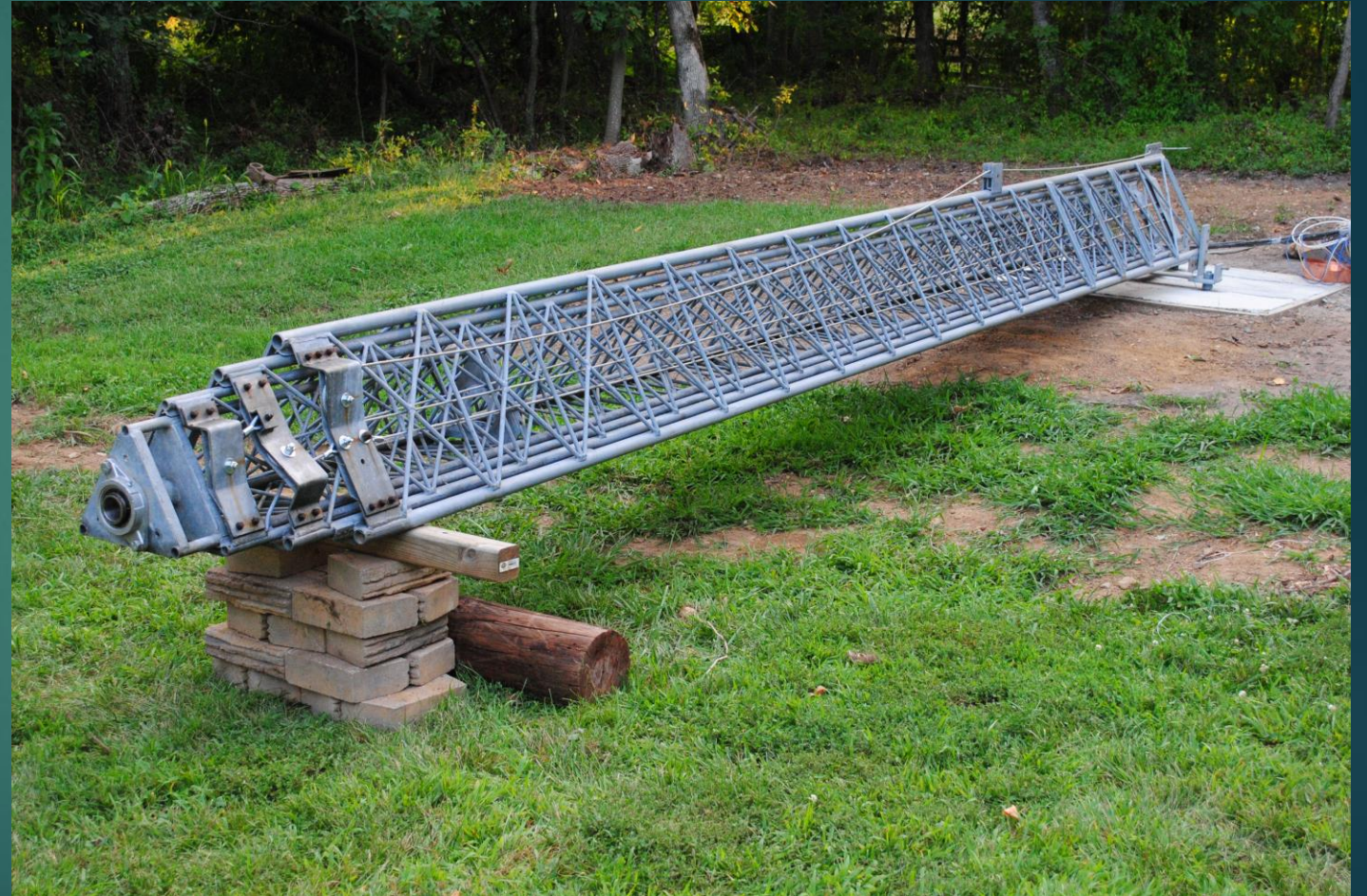
In Place Ready for Antennas
